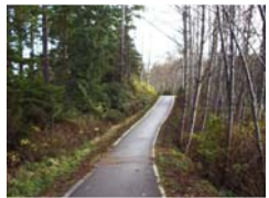
Buffering. Native plantings can provide a pleasant buffer between the MUP and the highway.
