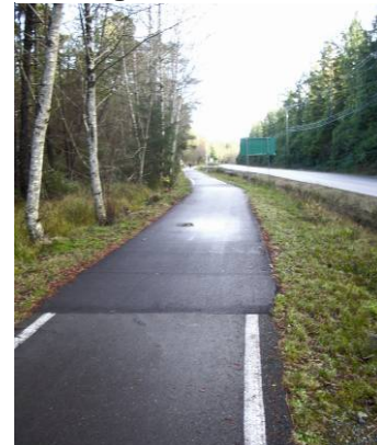
Figure 36: Where new pavement is installed ensure pavement markings are retraced
