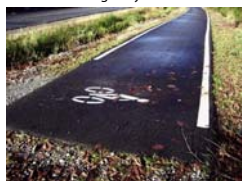
Reflective pathway markings. Iridescent paint increases visibility without contributing to light pollution.
