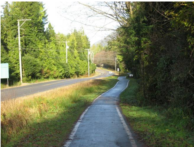
Figure 1: Existing Multi Use Path
