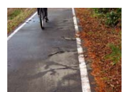
Path degradation - tree root damage.
